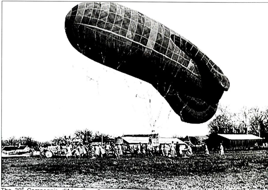
The 39<sup>e</sup> Compagnie d'Aérostiérs Caquot balloon, about to start on an operational flight. The observer is in the nacelle and the automobile winch can be seen on the left. Marcel Gogien
